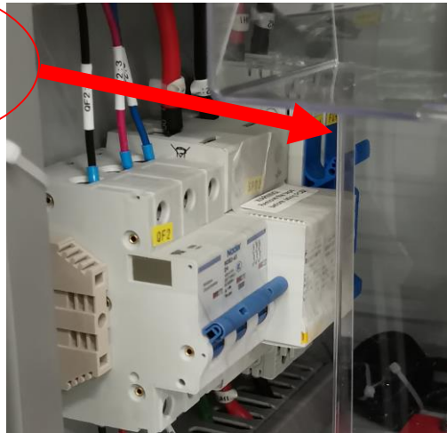
Figure 40. Remove the adhesive tape on DC SPD
