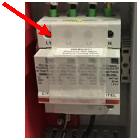
Figure 41. Remove the adhesive tape on AC SPD
