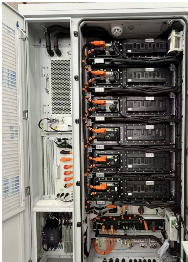
Figure 4-51 Internal cabinet connection cables
